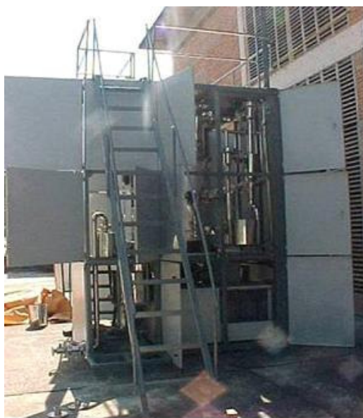
Figure 13. Indian gasifier installed at IPT Source: CENBIO, 2002
