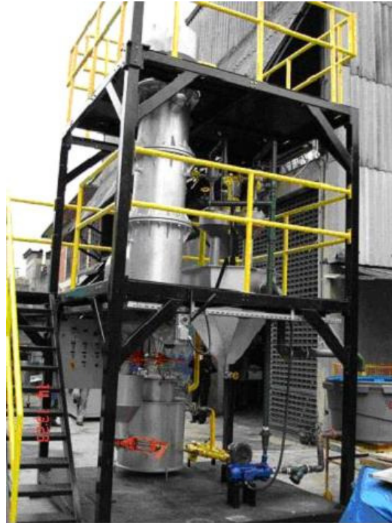
Figure 18. Gasifier of the GASEIBRAS project Source: CENBIO, 2003a
