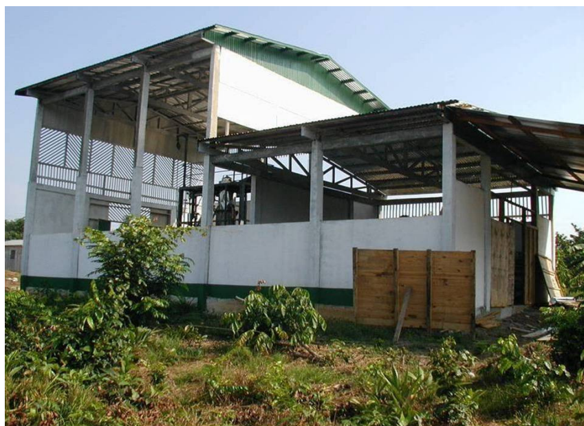
Figure 15. Shelter of the gasification system Source: CENBIO, 2002
