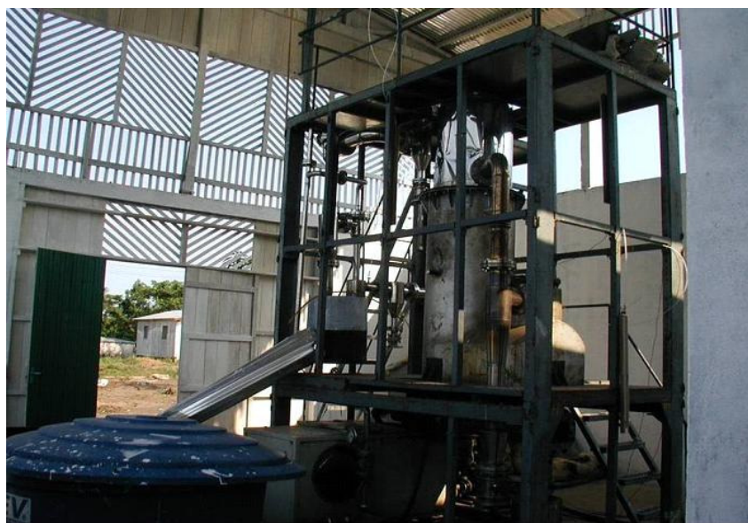
Figure 16. Gasifier installed in the community Source: CENBIO, 2002
