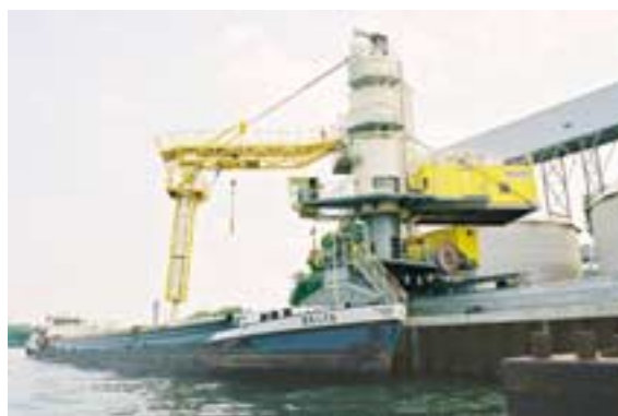
Unloading facility at the Amer Power Plant in the Netherlands. (Courtesy Essent, the Netherlands)
